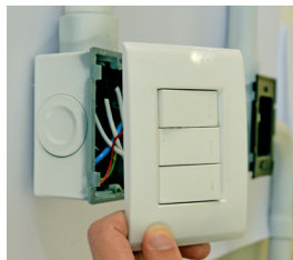
Figura 1 - Retire o interruptor
